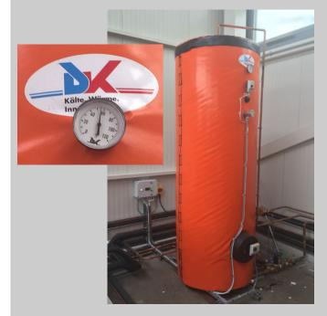
Heat re-claim: Our refrigeration plants feature an energy reclamation system which harvest the heat that would normally be rejected via condensers The reclaimed energy will be applied to heat the hot water
